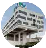
Hospital South Gai Gon VIETNAM
